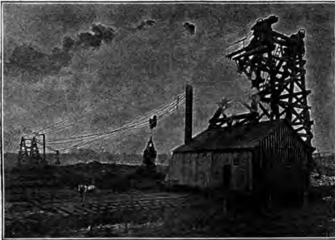
Fig. 113. Duplex Cableways Used on Hennepin Canal, Operating Two 1\frac{1}{2} -cu.-yd. Orange Peel Buckets.
